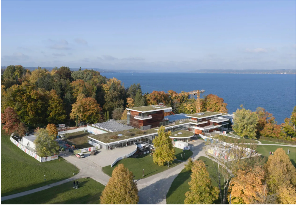
Construction Progress at the Buchheim Museum Extension, 2025
