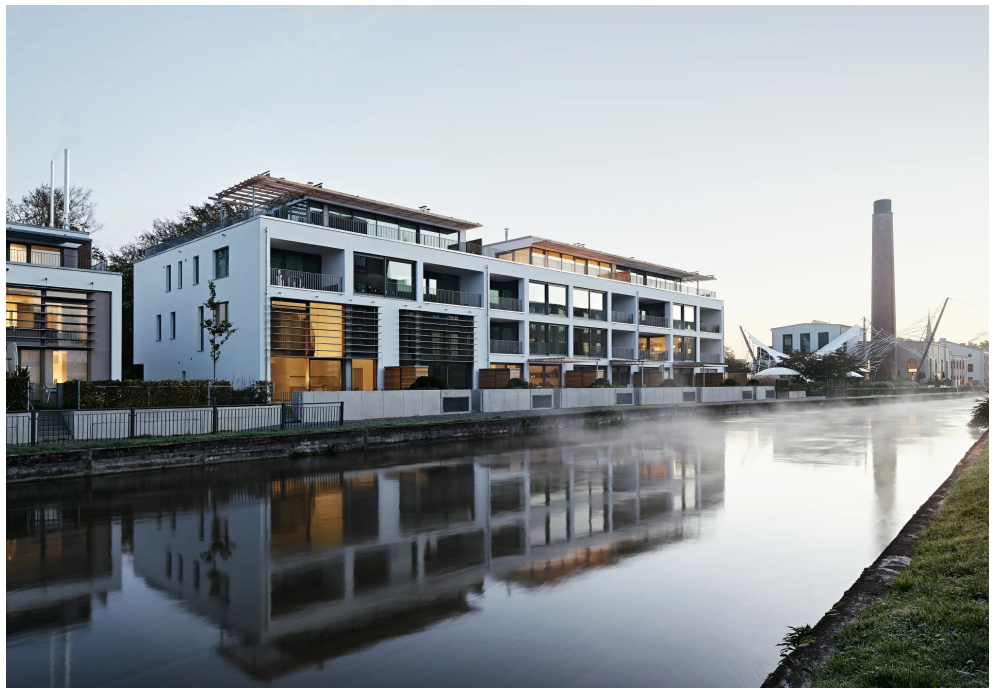
Apartment Building at the Rosengarten
